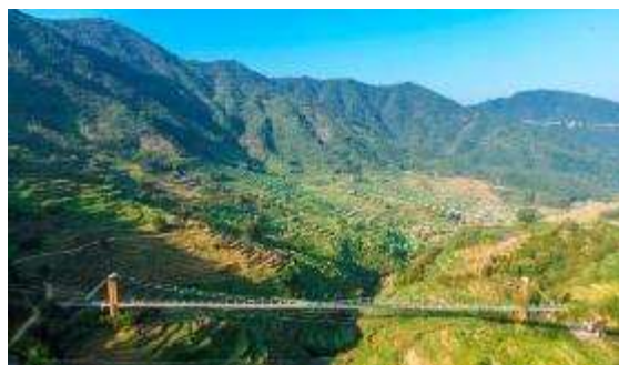
Wuyuan Glass Bridge
